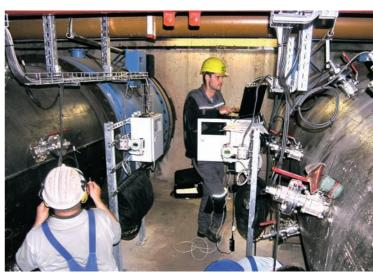
transducers contain neither electronics liable to drift nor mechanics subject to wear. According to the manufacturer, this guarantees the immensely important lasting reliability regarding the monitoring of the cooling water supply.
